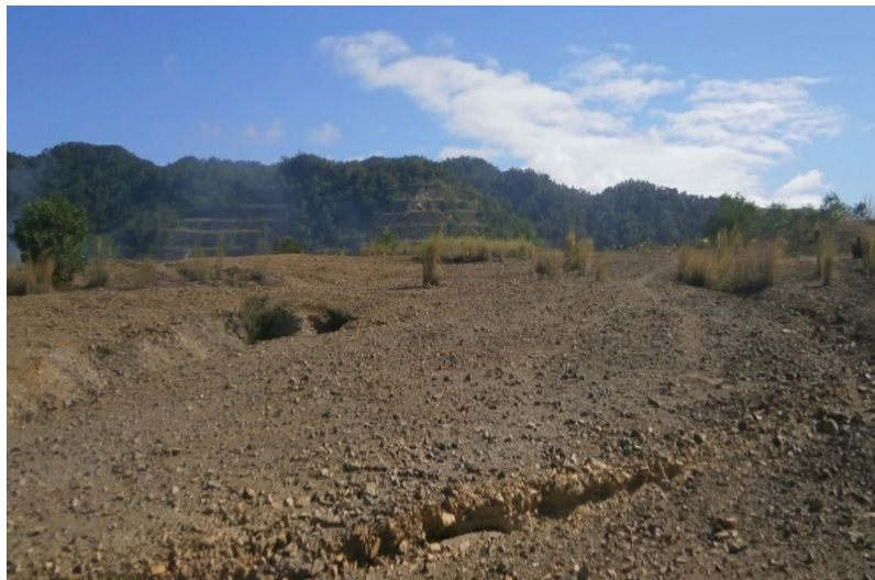
Fig. 3. Vegetation cover of the unrehabilitated area (area without intervention) located at the top most part of Consolidated Mines Incorporated (CMI) rock dumpsite in Mogpog, Marinduque, Philippines. February 15, 2016 (Photo credits: Katrine Mae B Mante).
